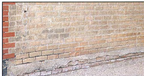
Repairing damaged masonry (like above) can be achieved by repointing the mortar joints. Look for evidence of deterioration such as loose bricks, cracks in mortar joints or damaged plasterwork. The new mortar should duplicate the period mortar in terms of strength, composition, colour and texture.
