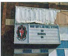
Can sign to be replaced and damaged transom to be repaired.
