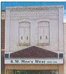
Three examples of diminished historic character resulting from removal or covering of original windows: KW Men's Wear upper storey windows, Hursts five bay windows, and Anavets ground floor and upper storey windows. Research is required to determine original window design for restoration.
