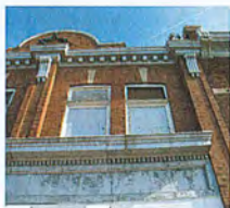
Window frames and lower level cornice, to be painted and repaired.
