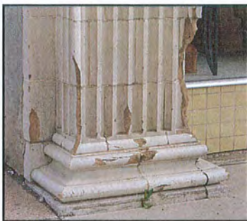
Deteriorated pillar base (above) requires repair/ replacement.
