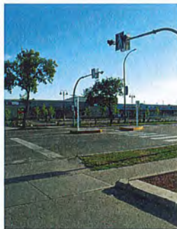
Crosswalk at Maple Avenue with overhead flashing pedestrian signals and refuge island in TWLTL.
