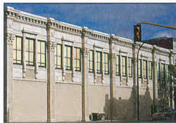
Three examples of diminished historic character resulting from removal or covering of original windows: KW Men's Wear upper storey windows, Hursts five bay windows, and Anavets ground floor and upper storey windows. Research is required to determine original window design for restoration.
