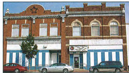
Three examples of diminished historic character resulting from removal or covering of original windows: KW Men's Wear upper storey windows, Hursts five bay windows, and Anavets ground floor and upper storey windows. Research is required to determine original window design for restoration.
