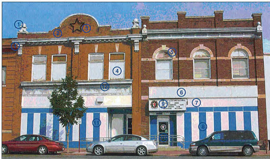
Contemporary photo of the Anavets illustrating the devalued historic character resulting from the removal, covering, or physical deterioration of the architectural features. The numbers correspond with a description of the various building features.
