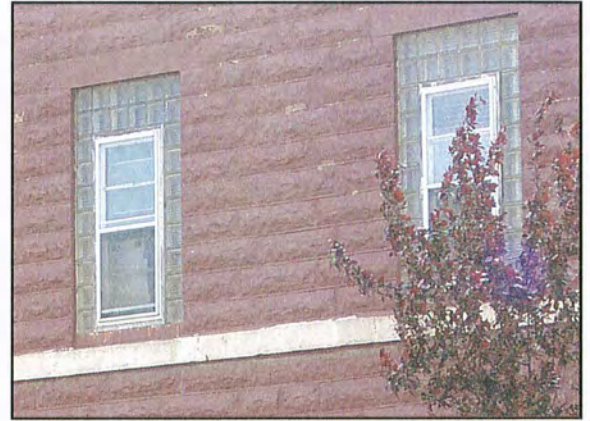
Windows (above) have been slightly altered; the openings are partially blocked. Typically, this should be avoided and window assembly authenticity should prevail.
