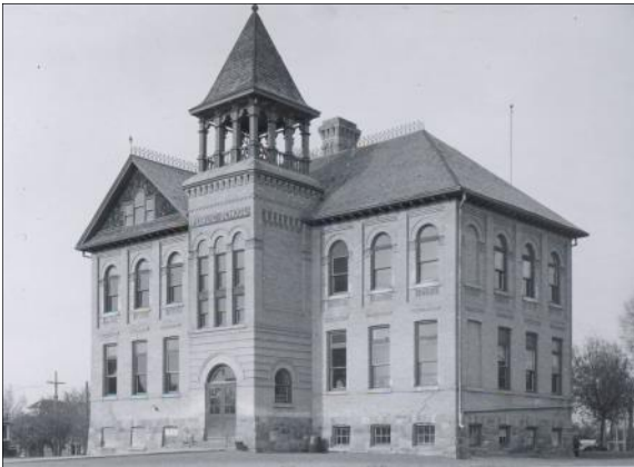
Victoria School built in 1899 on the present site of Shaw Park
