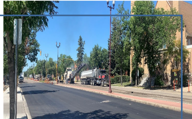
Smith Street Paving
