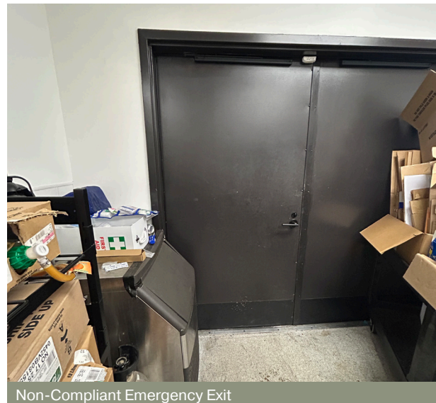
Non-Compliant Emergency Exit
