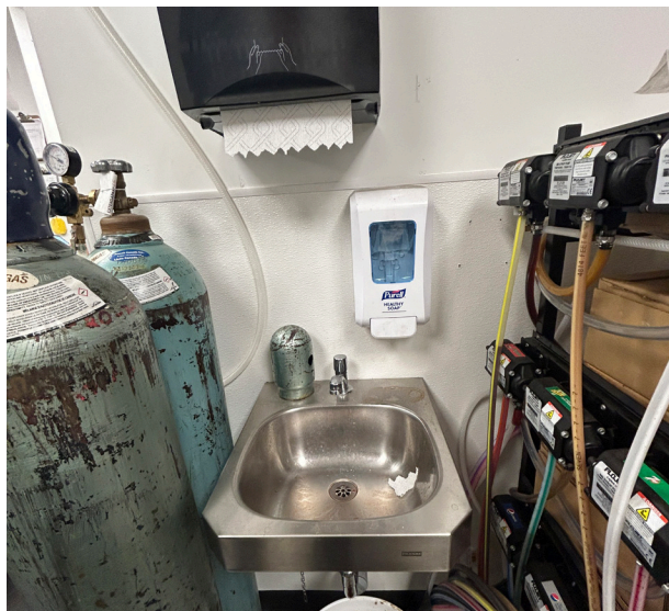
Handwash Sink - Impeded
