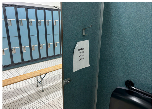
Accessible Stall Coat Hook and Latch
