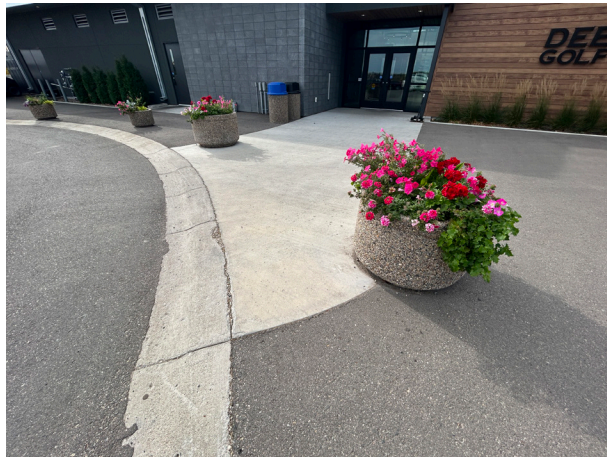
Curb Cut from Parking to Pathway
