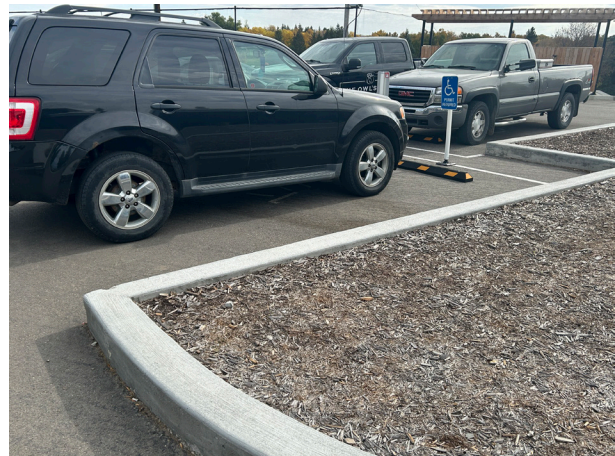
Accessible Parking Stall - No Curb Cut
