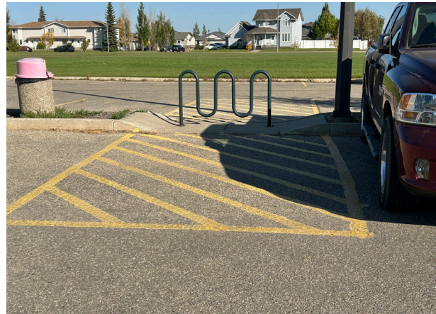
Exterior Pathway Impeded by Bike Rack
