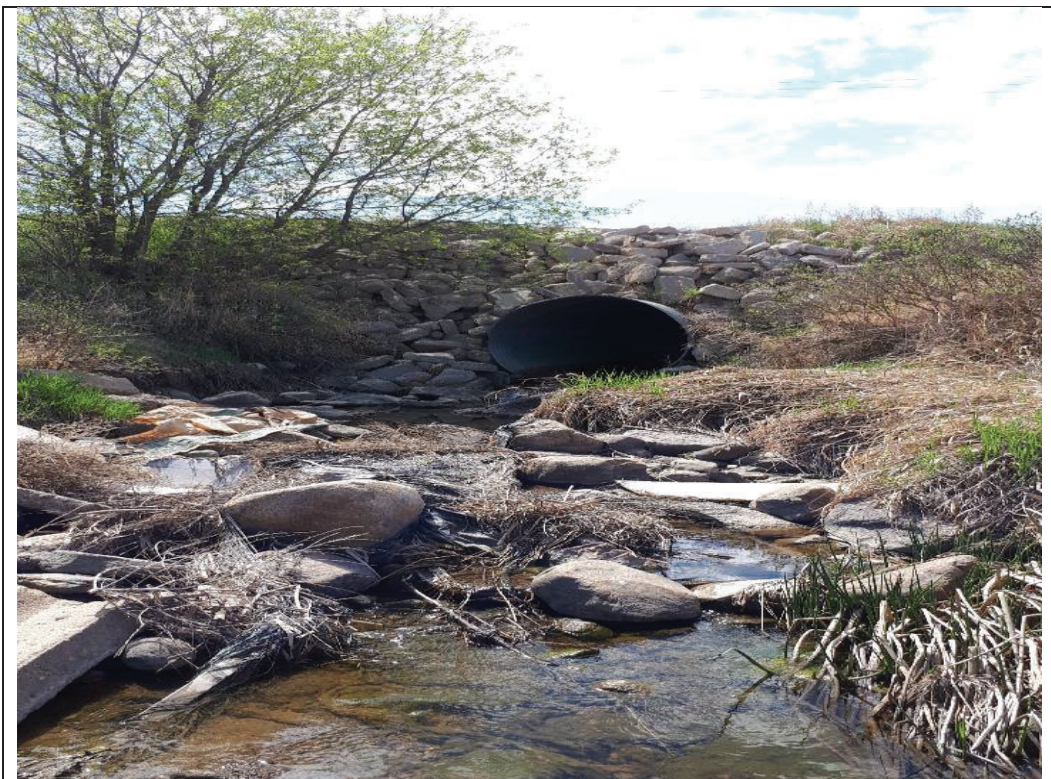
Photo 10. Looking upstream at the culvert at the southwestern limits of the Project Location.
