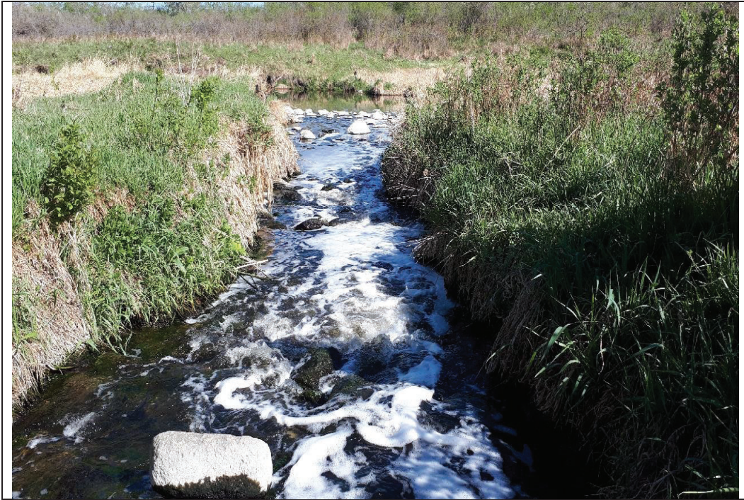
Photo 7. Discharge effluent channel, looking downstream at main reach of Yorkton Creek.
