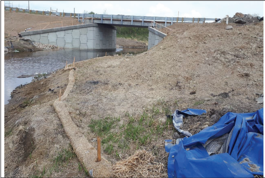
Photo 1. Standing on right bank, looking upstream at the Vehicular Bridge constructed.
