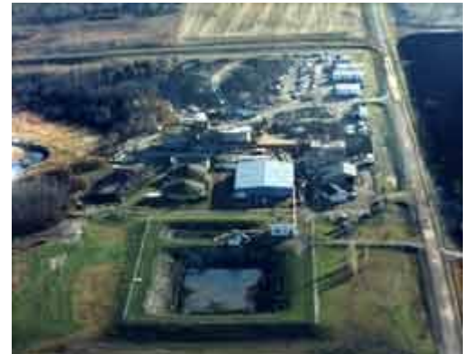
Current plant under construction. 1990
